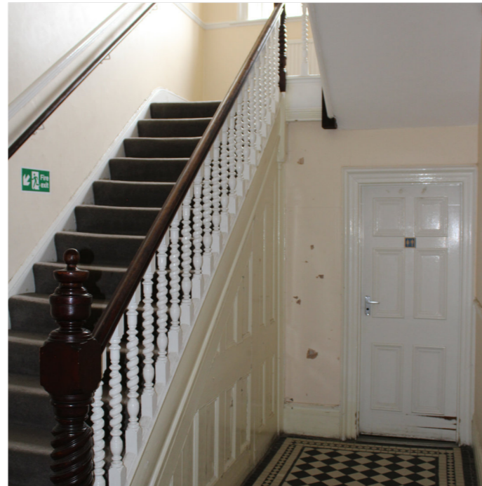
STAIRS AT GROUND FLOOR LEVEL
