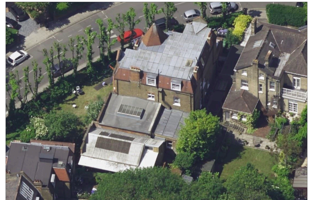
DETAIL LOOKING WEST
